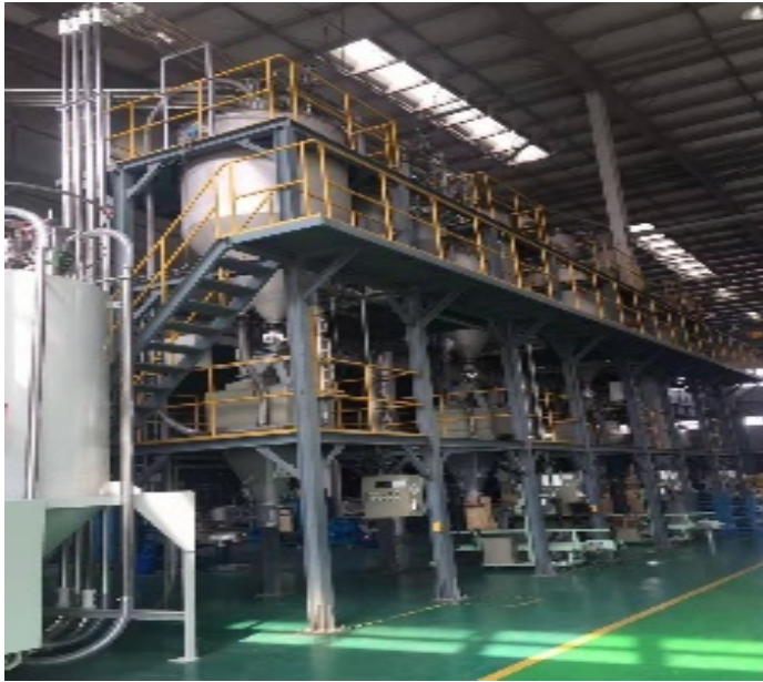
Plastic Injection & Molding Pilot Plant
